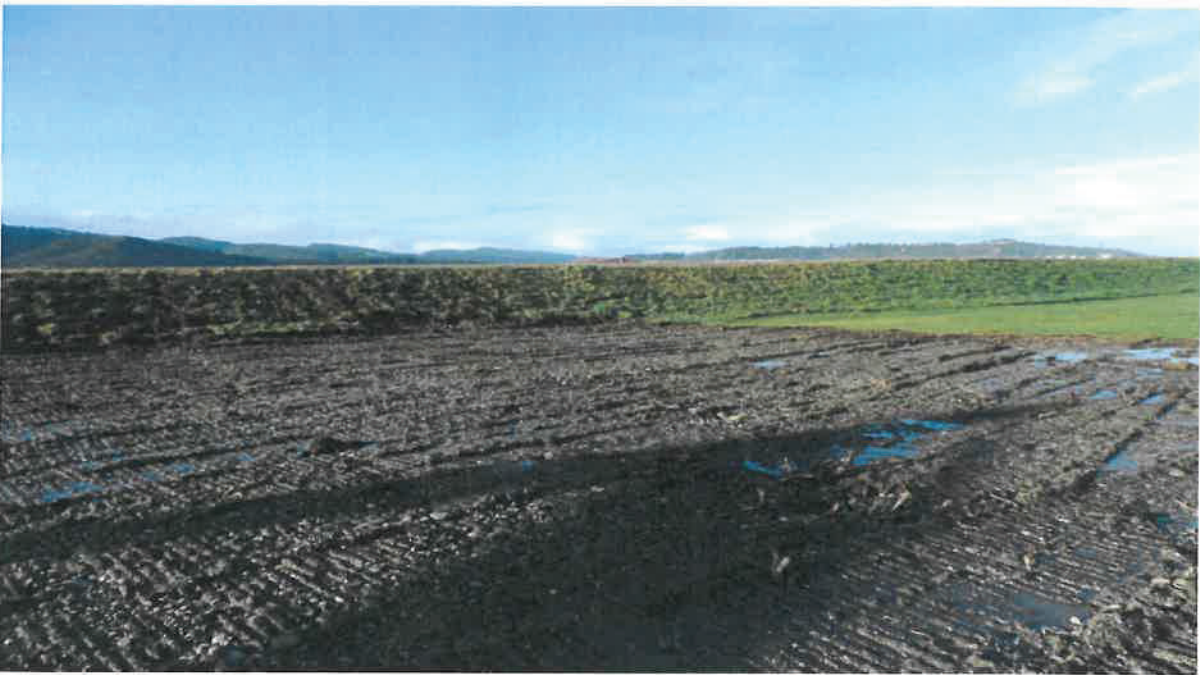
Completed works, Re-grassing will be undertaken in Spring.
