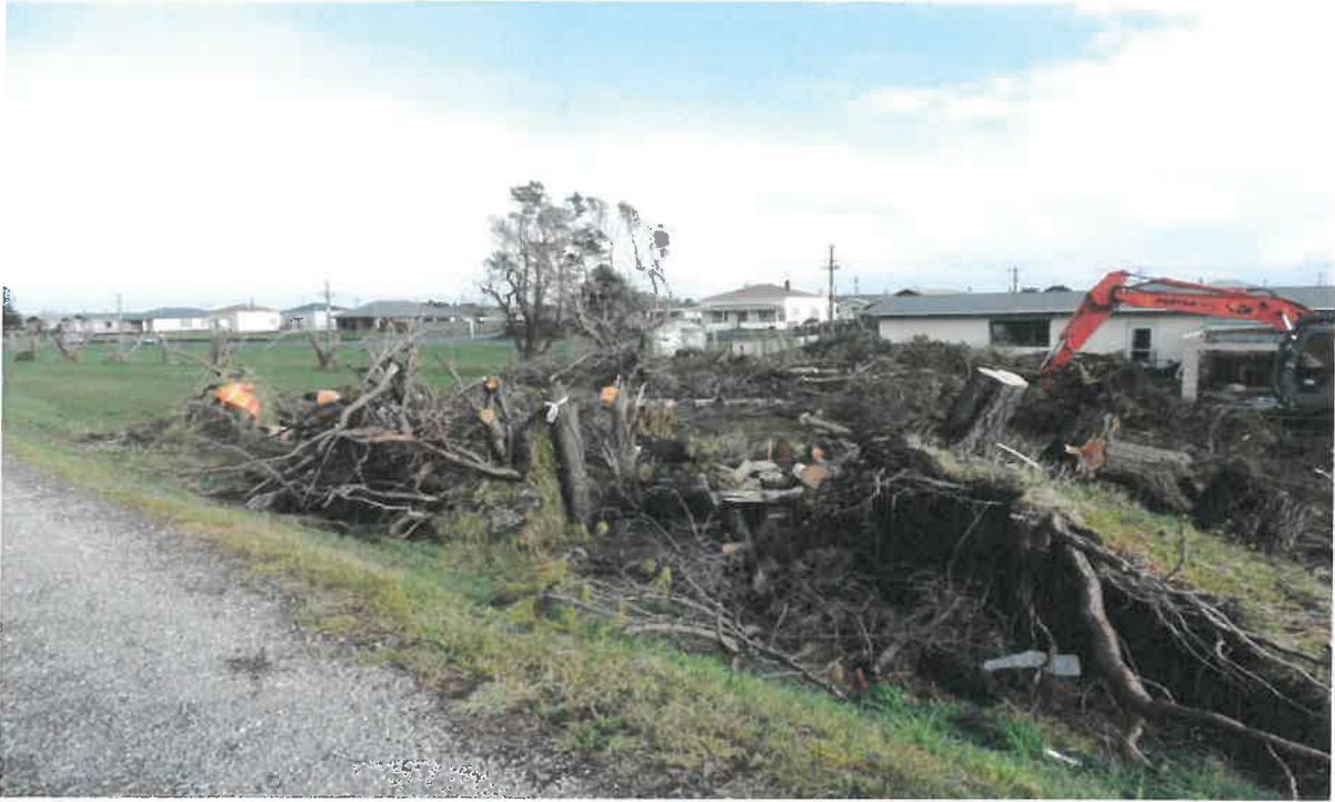
Cutting up and disposing of trees behind the Scout Lodge
