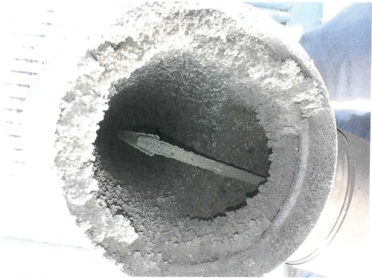
An Oeko Tube device installed inside the flue of a coal fire, Reefton
