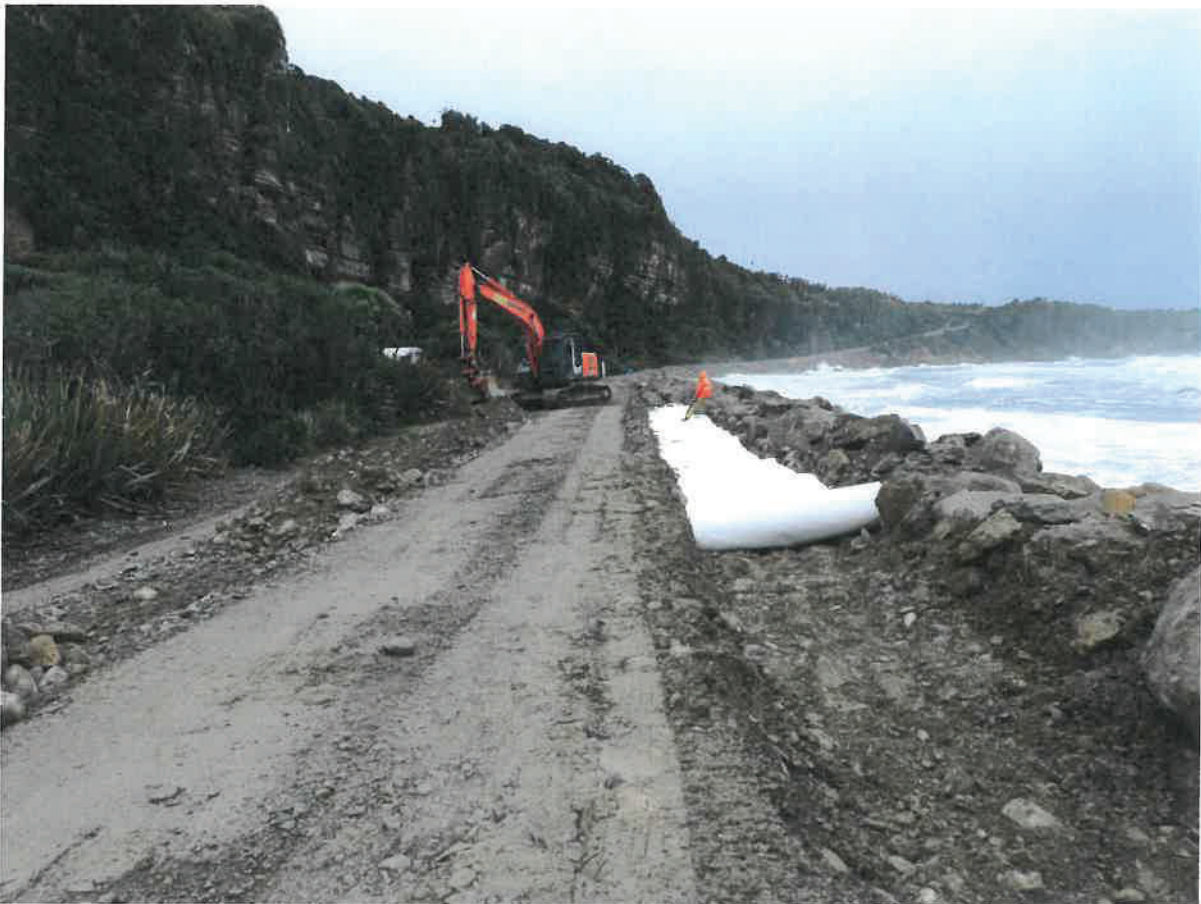
Punakaiki Seawall – Maintenance Construction – July 2014
